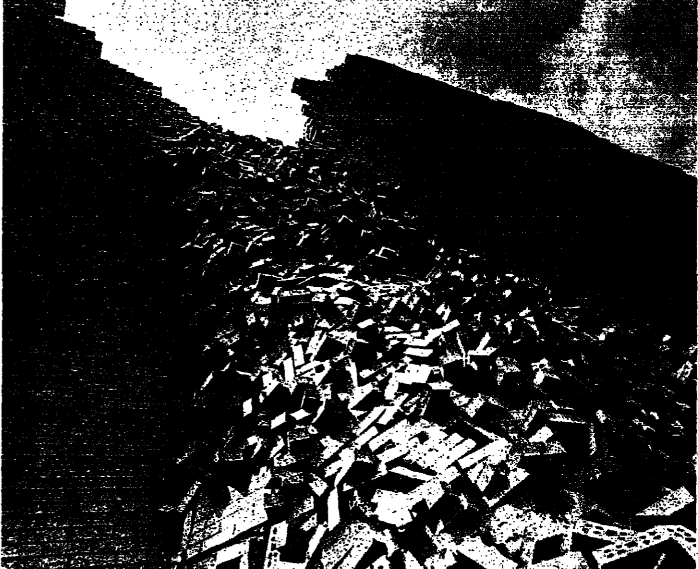
Loose bricks spill down the facade (on purpose) of the Best Products Store in Houston, Texas.
